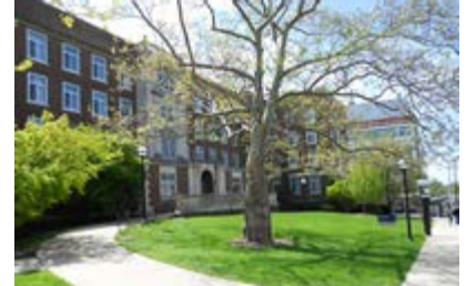
Couzens Hall: ASHRAE +30% and Designed to Earn the ENERGY STAR® certification
