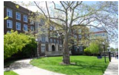
Couzens Hall: ASHRAE +30% and Designed to Earn the ENERGY STAR® certification
