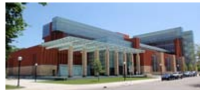
Ross School of Business: LEED-NC Silver
