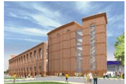
Michigan Stadium Renovation and Addition
