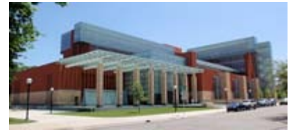
Ross School of Business: LEED-NC Silver
