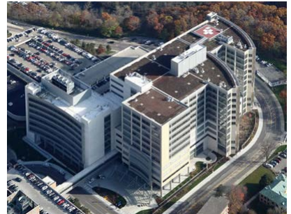
Mott Children's and Women's Hospital: Goal of LEED-NC Certification
