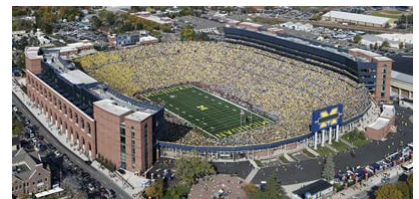
Michigan Stadium Renovation and Addition
