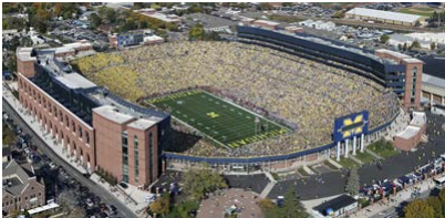
Michigan Stadium Renovation and Addition
