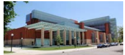
Ross School of Business: LEED-NC Silver
