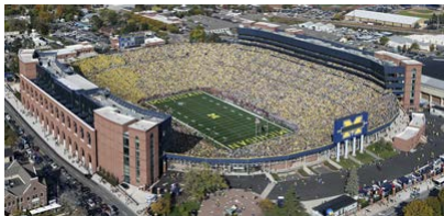
Michigan Stadium Renovation and Addition
