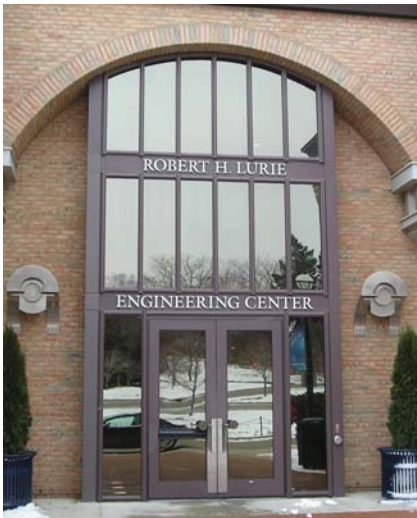
Example - building in totality - donor name on exterior, above entrance door, all upper case, 5" stainless steel letters
