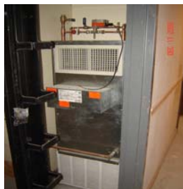
Telecomm Room – FCU Installation
