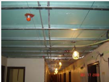
2nd Floor Corridor – Ceiling Installation
