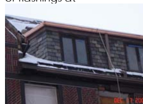
Copper Gutter Installation
