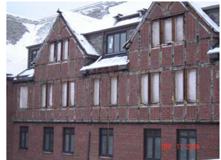
5 Side (North) Elevation – Half Timber Removal
