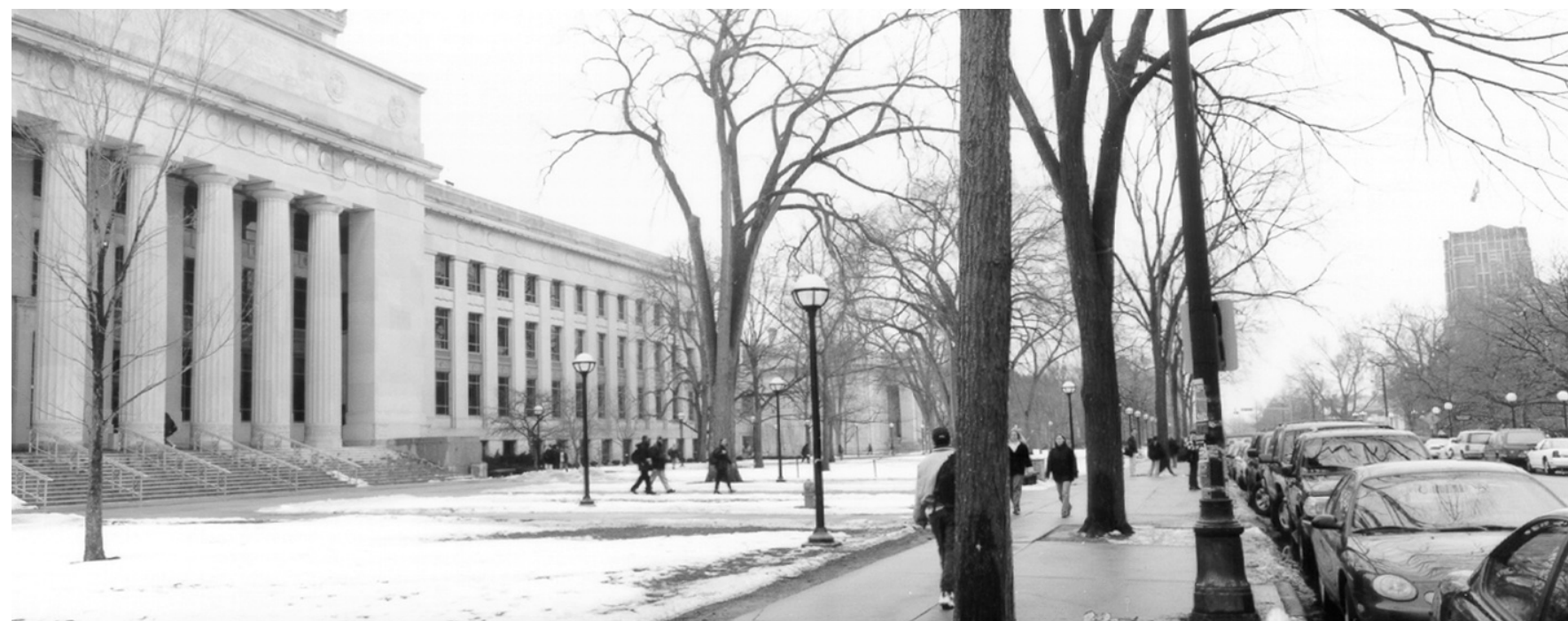
fig. 2. View of Angell Hall along State Street
