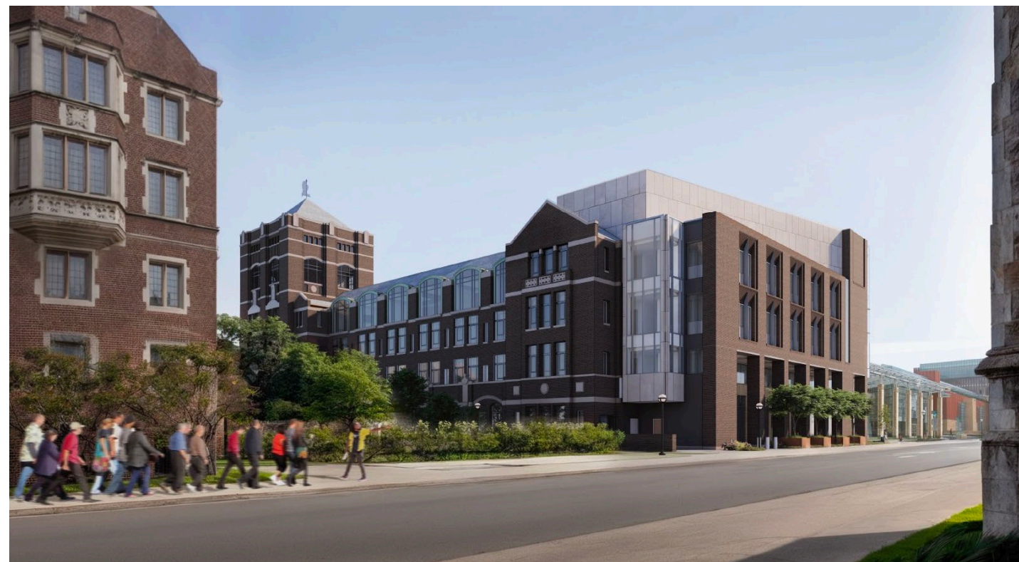
View of West (Tappan) and North Elevation
